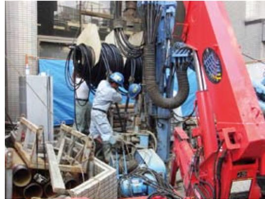
Retrofit of GHP system to an office building in central Tokyo: inserting U-tube (Sasada Building)
