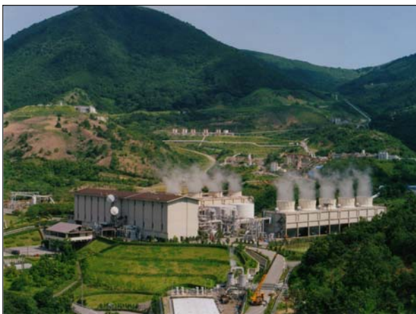
Kyushu Electric, Hatchobaru Power Station. Two phase flow transmission, double flash 2x55MW, No.1 unit operation started in 1977.
