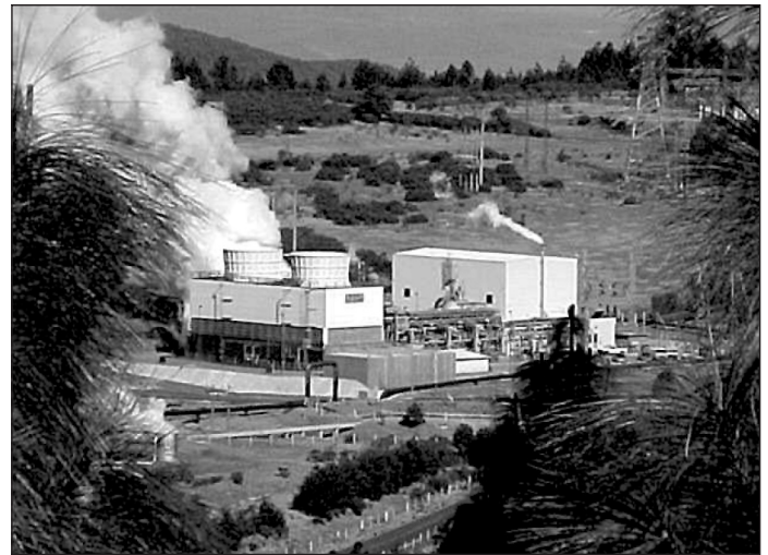
One of the four 25-MWe units of the project Los Azufres II
