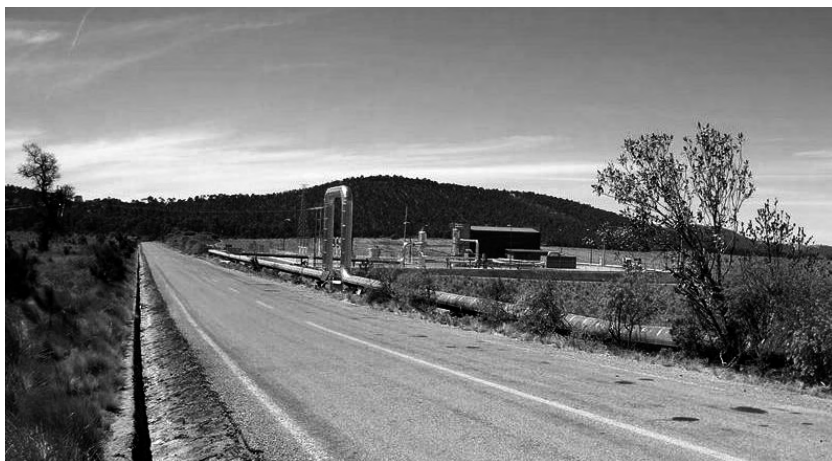
View of Unit 8 and its steam-pipe in Los Humeros
