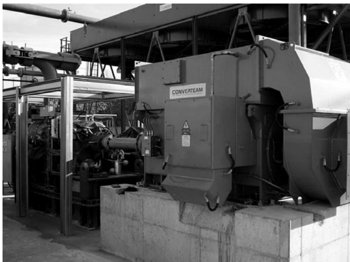
Figure 1. The Soutz ORC power plant: installation of the generator
