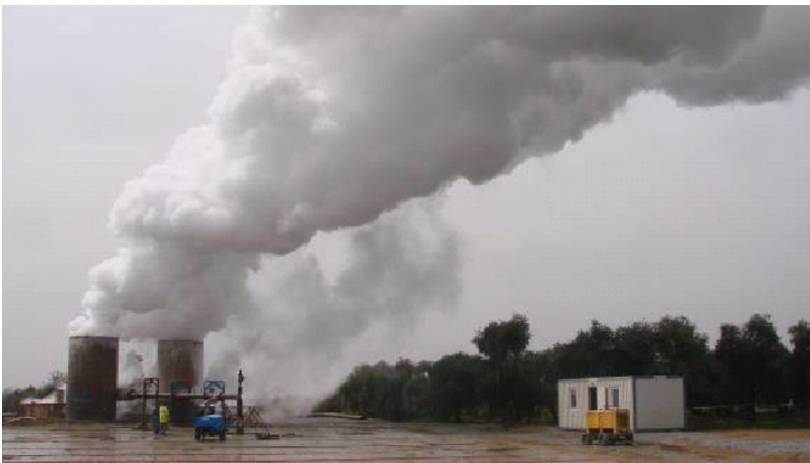
Fig. 3. Testing of a production well
