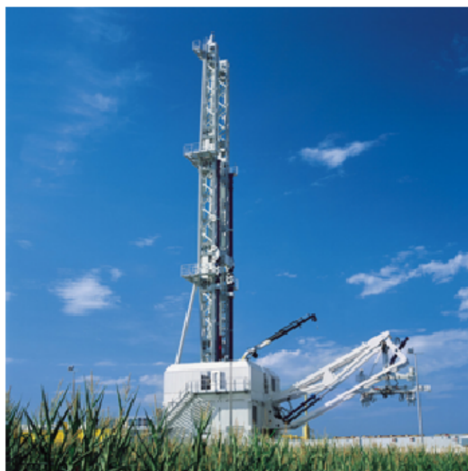
Figure 3: The first deep drilling rig of the TI-350 type
