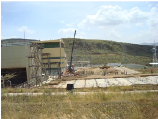
Olkaria II, Unit 3 (35MW) construction works in progress
