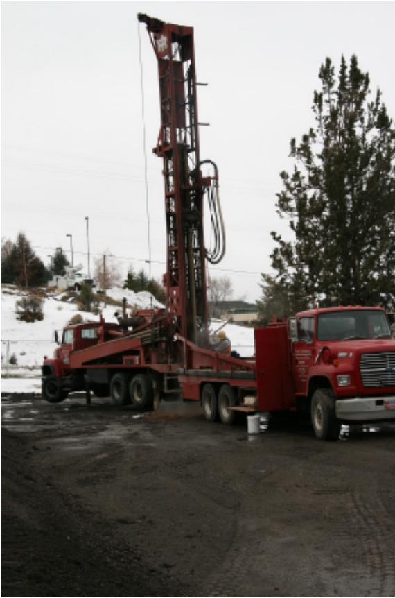
Start of drilling for surface casing
