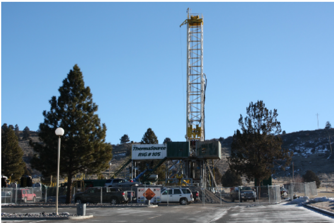
The drilling rig being set-up.
