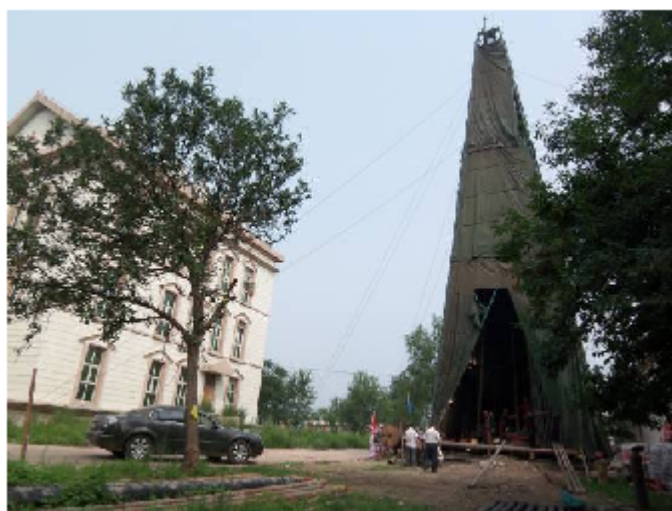
Figure 2: Drilling for hot water in Yanqing County
