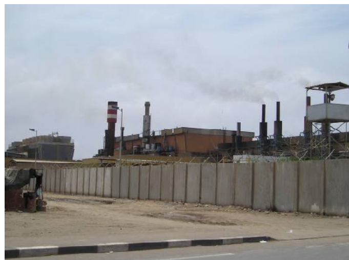
Figure 1: Boulaos thermal power station, Djibouti.
