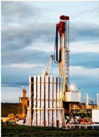
Trailer-mounted, highly automated DrillMec HH300.
