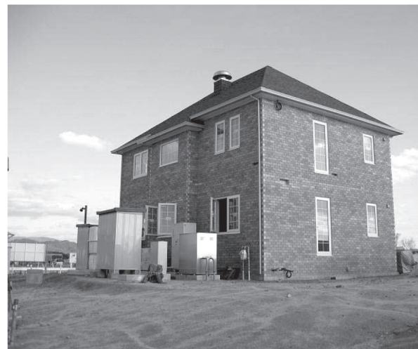
Fig.3 An experimental house constructed on reclaimed land in Fukuoka city, Kyushu, Japan. It is made of brick and is a standard 2-storey house for a family of four.
