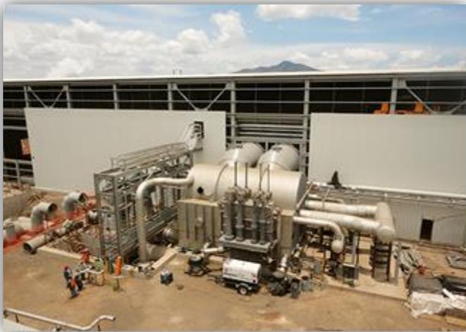
According to SPX Heat Transfer, ADCC is a licensed technology designed for geothermal power that condenses steam directly from geothermal wells or steam flashed from hot brine. It uses a turbulent film to condense the steam. The higher thermal efficiency of the ADCC technology has many benefits and saving features like:
