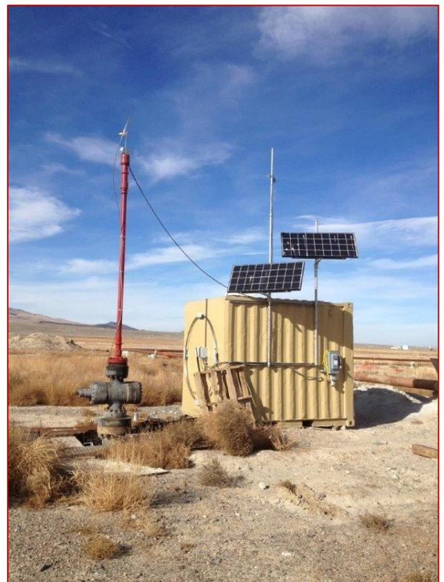
*The RRG-9 ST-1 wellhead fitted with a lubricator. A distributed temperature sensor was run through the lubricator to measure well bore temperatures. (Photo: GTO)*
