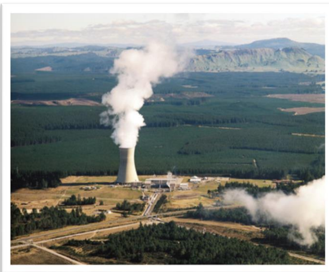
View of the Ohaaki's 105 meter-high cooling tower. Using natural convection, the tower cools the water used to condense the steam as it exits the power turbines. Photo credit: © GNS Science / Science & Society Picture Library.
